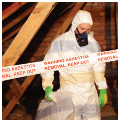
Sealing a plastic rubble bag of asbestos
