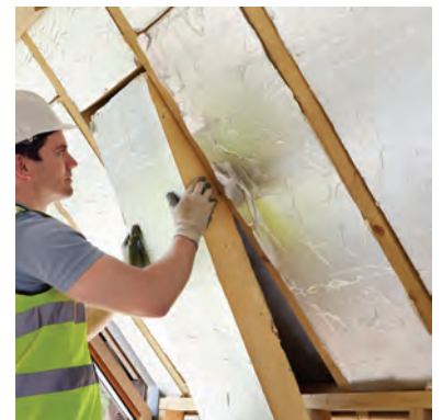
Taping rigid foam insulation joining & splicing
