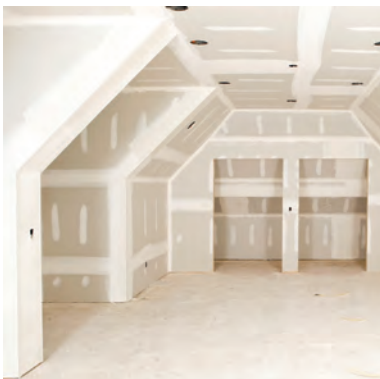
Corner plasterboard joints
