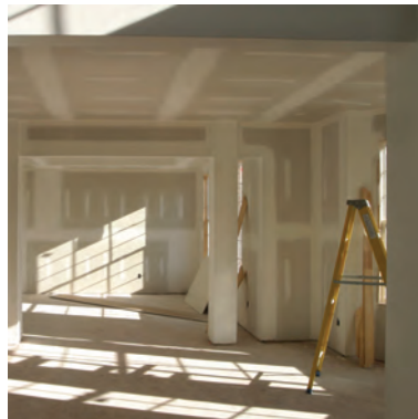
Ceiling plasterboard joints
