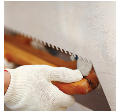
Repair cracks in plasterboard walls
