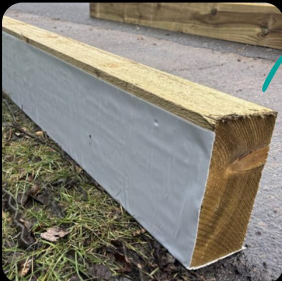
Position the bottom sleeper, which rests directly on the ground, with tape along the bottom and on the interior face of the sleeper bed. All subsequent sleepers should overlap by 50 mm to ensure moisture cannot seep through.
