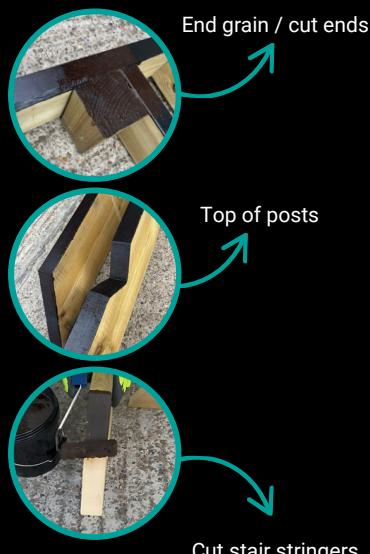
End grains, tops of posts, notches, noggins and wall plate / ledger boards quickly absorb moisture, leading to rot, decay and premature failure. While the right tape is the proven solution for joist tops, it can be difficult or impractical to apply on these awkward details. HD Timber Coating is designed for those hard to tape areas.
