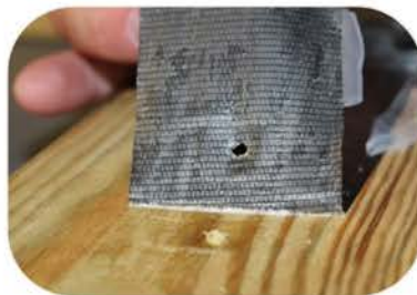
Complete seal around screws
